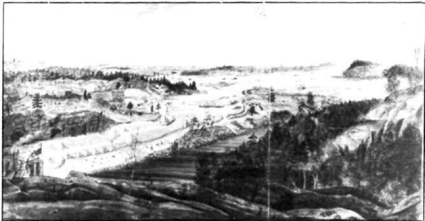
Construction at Kingston Mills; work on dam in progress in centre background; the steamboat 'Pumper' at the far left was used to drain water flooding the lock pits; Burrowes Sketch, Archives of Ontario
