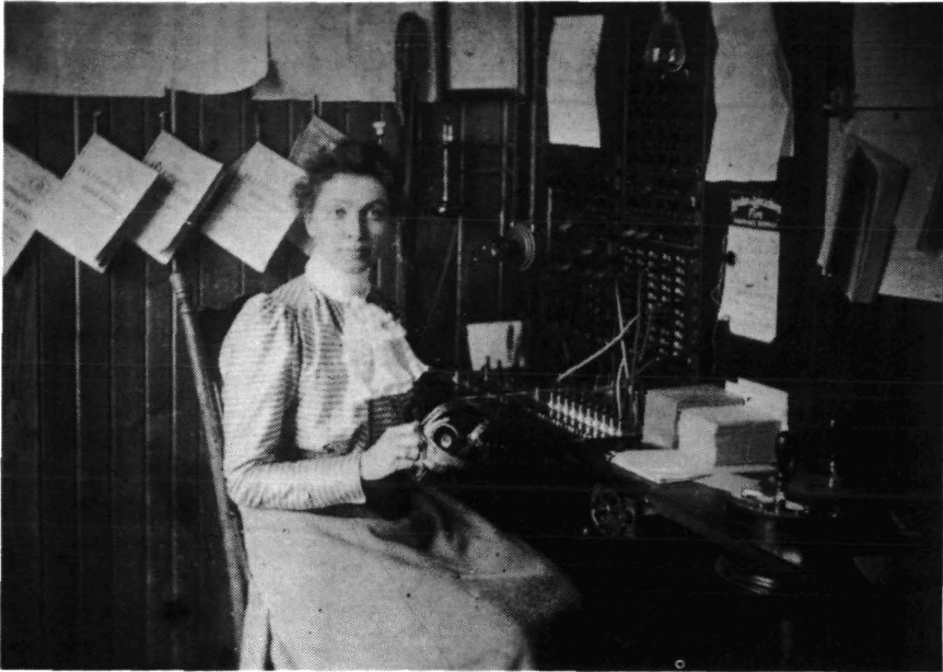
Miss Ida Gardner, At No. 1 standard switchboard. She was the first operator in Winchester, Ontario, 1897. (Photo #13720 Courtesy of Bell Canada Telephone Historical Collection)
