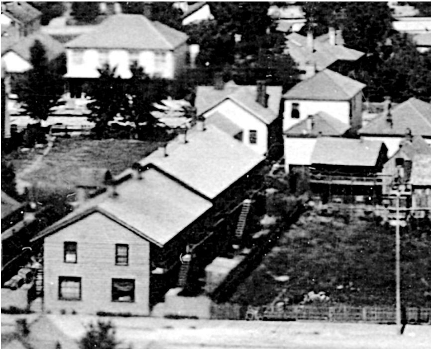
Figure 7: Tenement block at 132 Johnson Street, c. 1891. Detail of Image A-03384, courtesy of Royal BC Museum, BC Archives.
