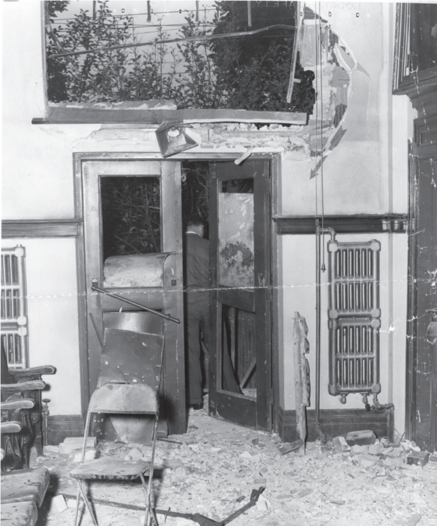
A close-up of the damage, n.d. © Government of Canada. Reproduced with the permission of Library and Archives Canada (2022). Royal Canadian Mounted Police fonds, vol. 2623, access request A-2015-00092, Library and Archives Canada.
