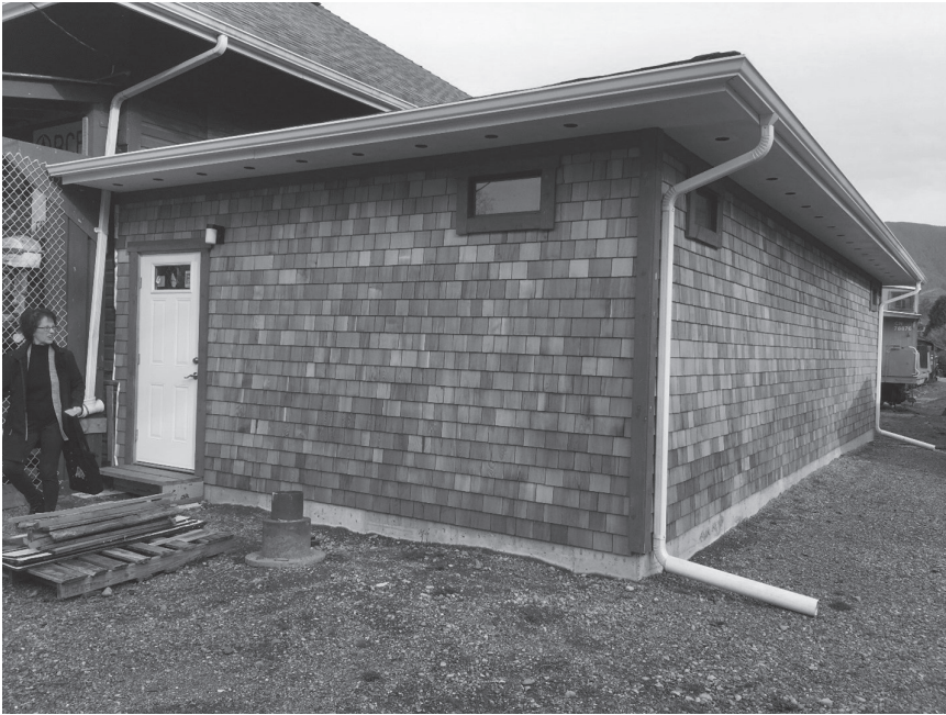
The IWA Annex almost completed, 2019.
